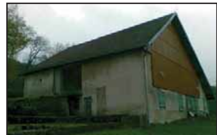
Figure 32: Point Pt1 (865m)
