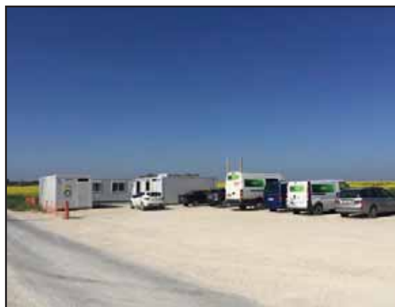
Figure 5: Base de chantier
