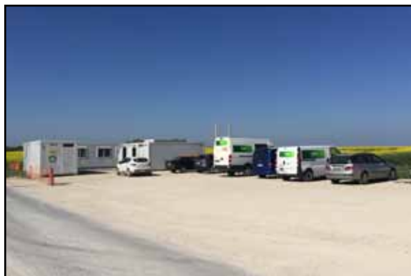
Figure 5: Base de chantier
