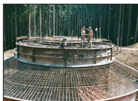
Figure 247: Installation du coffrage
